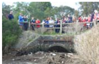
The end of a drain
